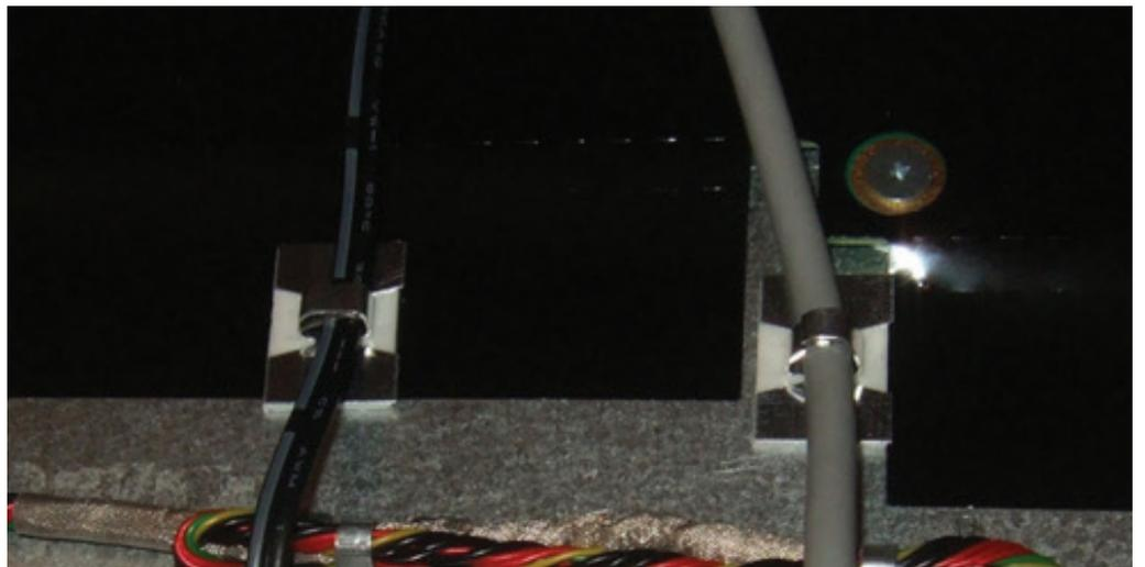
FIGURE 25 CABLE CLIPS HOLDING CABLES IN PLACE
